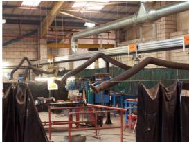
Extraction Rails are an advantage when working over a huge workspace on large items. Each exhaust arm is attached at a height of three metres and is rotatable through 360° due to its positioning on the rail. This gives the operator a free and unobstructed working area. In addition the arms are able to be moved to any point along the rail giving this workshop a floor area of 360m² covered by extraction.
